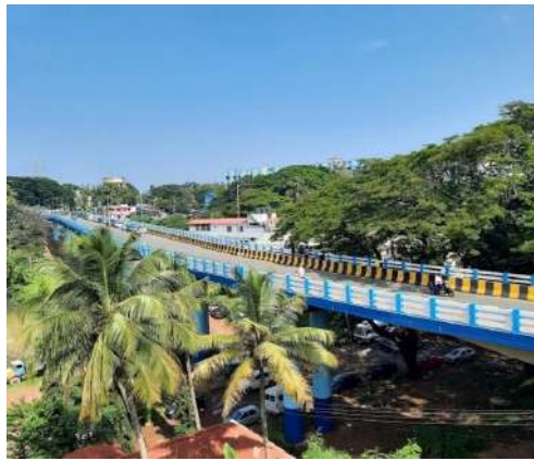
Figure 34. Flyover, GMC Thiruvananthapuram
