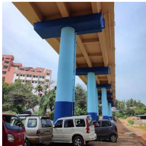
Figure 37 Flyover, GMC Thiruvananthapuram
