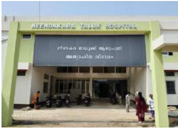
Front view of Hospital
