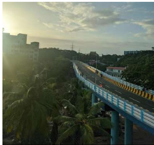
Figure 36 Flyover, GMC Thiruvananthapuram
