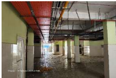
Inside common corridor area
